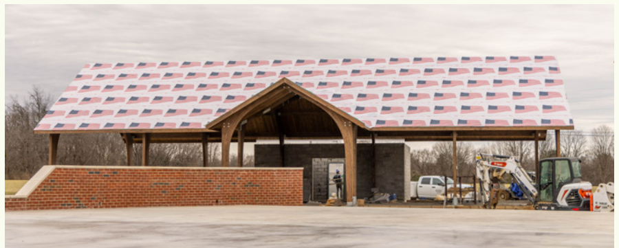
The park will feature a number of amenities for the public to use, including free public Wi-Fi, a large stage and a covered pavilion, shown, with restroom facilities. Though the patriotic underlayment is certainly eye-catching, a metal roof will be installed on top.
